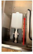
**Step 2:** To remove the soap dispenser slide it in an upwards direction.
